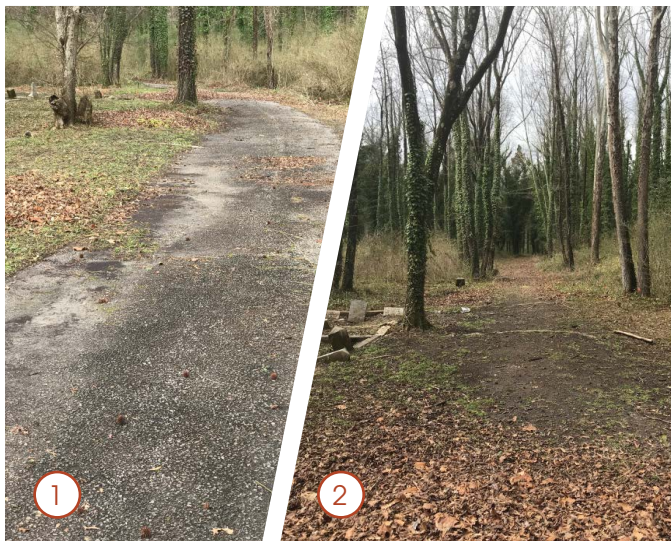
① Existing Lower Loop Roadway, eastern side
