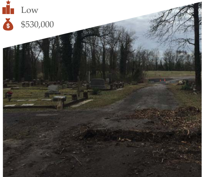
Interior Primary Roads
